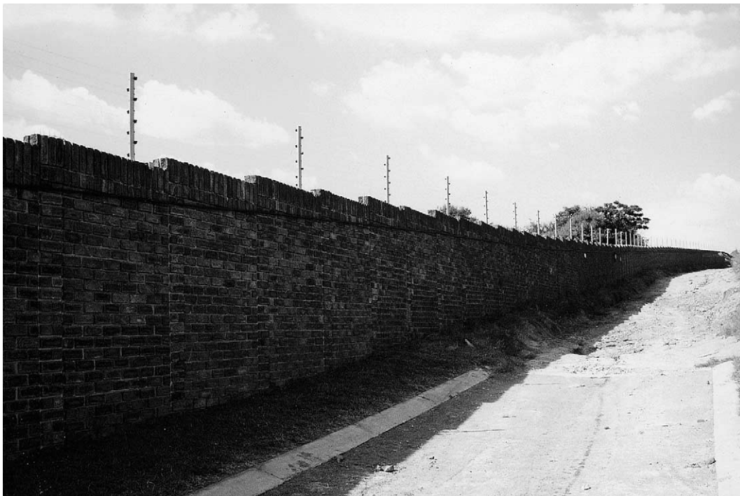
Fig. 2. Dainfern's electrified perimeter wall.
